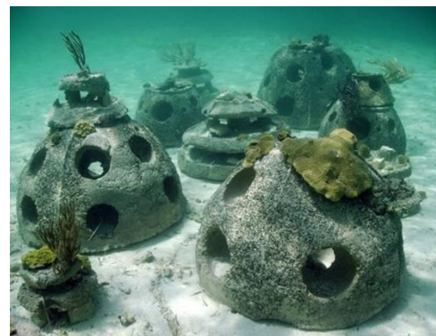
Figure 5. Example of concrete reef dome structures (Reef ball foundation, n.d.).
