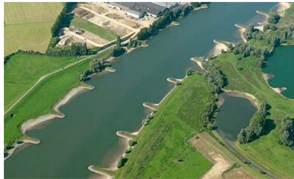
Figure 5.4: Example of groynes in a river to stabilize the channel and its banks. (Rijkswaterstaat)
